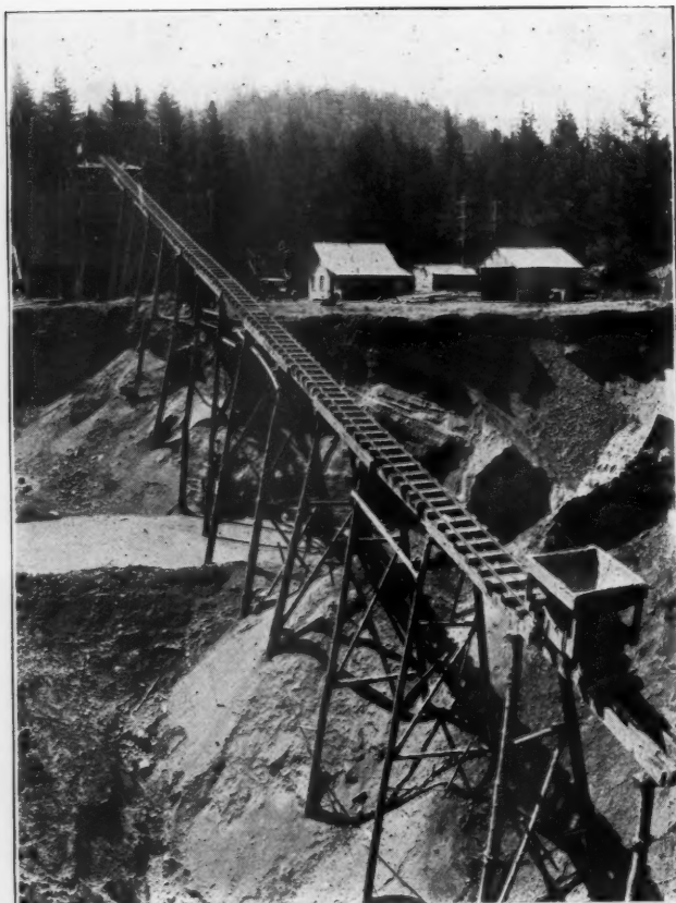
The Trestle Leading from Pit to Screening Plant and Storage Bins
